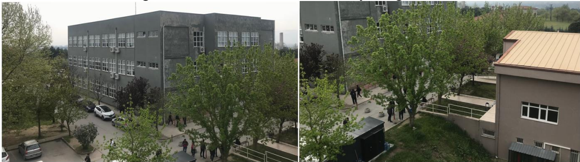
Figure 4. View towards classroom buildings
