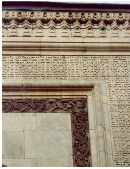
Picture 10. Amasya Bayezid Pasha Lodge, eaves line details
