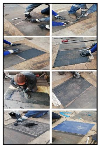
Figure 4. Images of belt splice preparation stages
