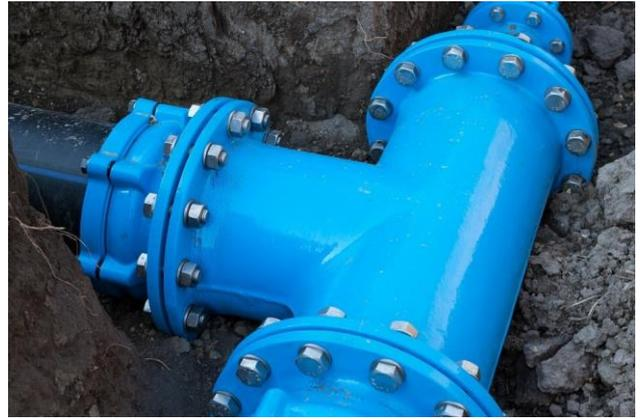
Figure 16. Bolt-on flanged pipeline system
