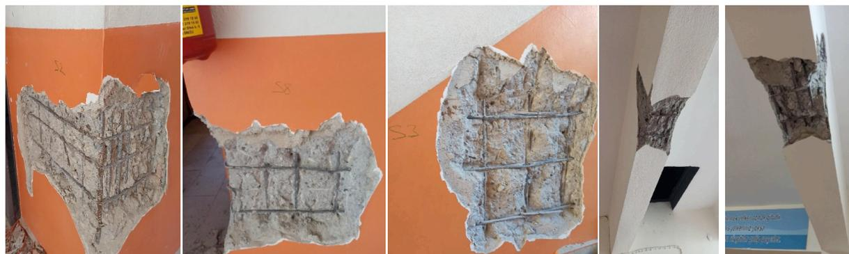
Ground SZ13 column    Ground-storey SZ16 column    Ground storey PZ05 shear wall    Ground K112 beam    Ground SZ27 beam
