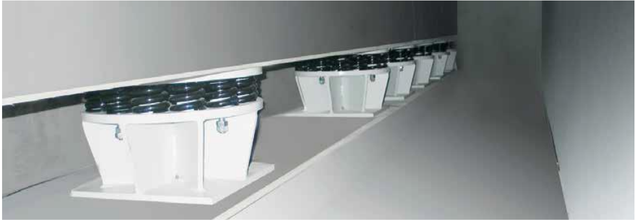
Figure 6. A typical spring system at the supports [10]
