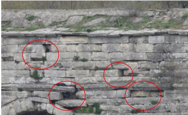
**Figure 6.** Damage and fragmentation in stone on façade of the Eğri Aqueduct [8]
