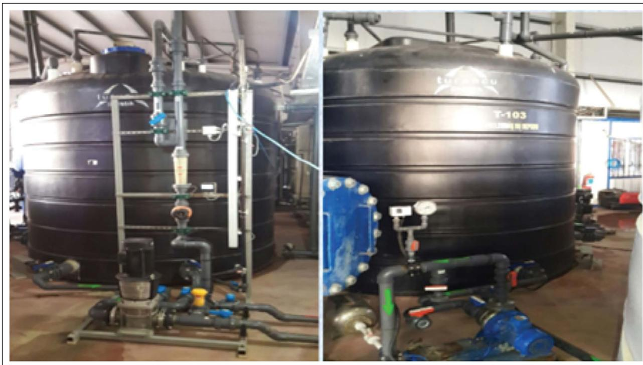
**Figure 5.** Tank 3 for pH adjustment.
