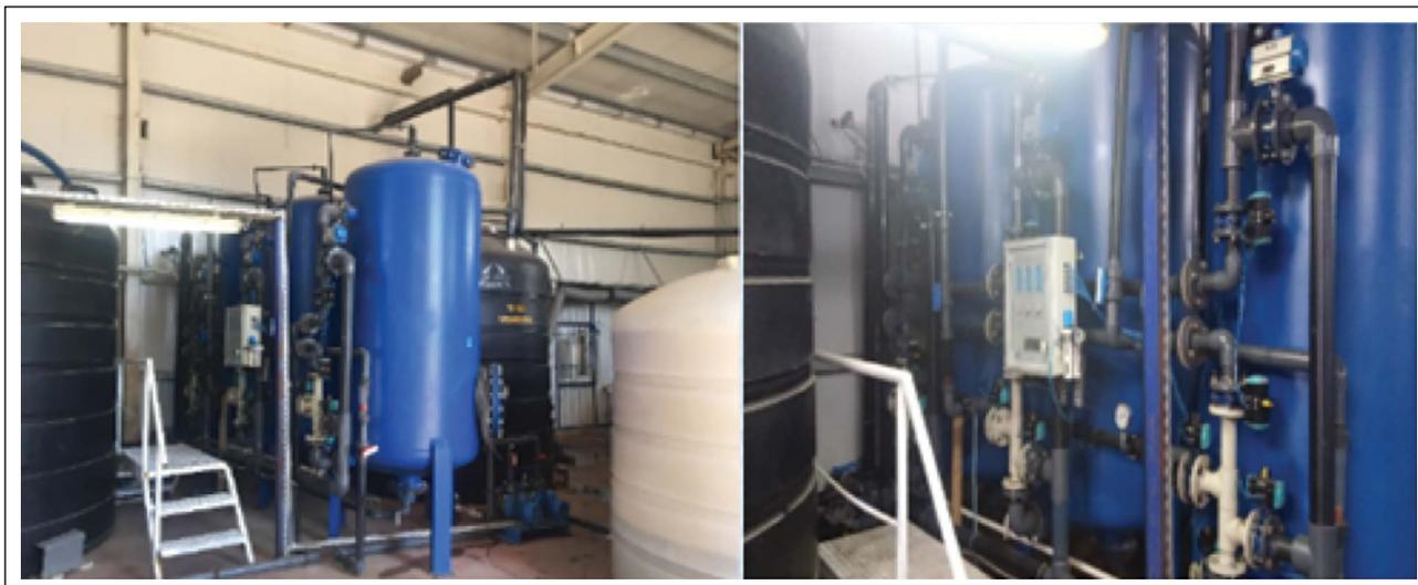
**Figure 4.** Sand filters in the system.
