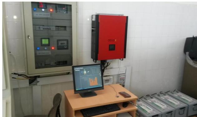
Figure 5. Control and recording system
