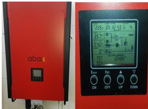
Figure 8. 3 Phase Hybrid Inverter
