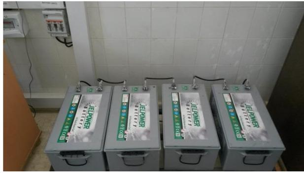
Figure 7. Batteries connected in series with 200 Ah 12 V
