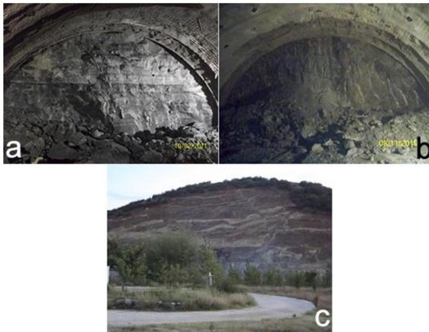
**Figure 4.** Geological units to be encountered in T35-GT2 (a: Porsuk Formation claystone, siltstone unit (Bozüyük) crossed at T35 b: Very weathered Bozüyük Granitoid passed through tunnel no 35 c: Cut with hydrothermal quartz and pegmatite veins in different thickness-position “Bozüyük Granitoid”(T35 entrance portal east section, highway cut)).
