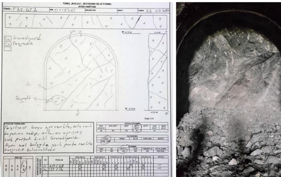
**Figure 7.** Tunnel face and geological map form of Bozüyük Granitoid region.
