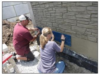
Figure 4. Stamping method on concrete surface
