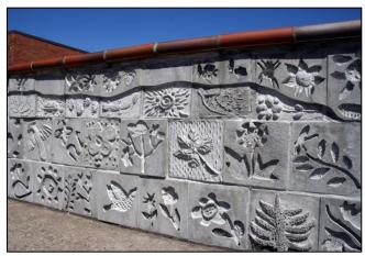
Figure 5. Positive and negative patterns on concrete surfaces
