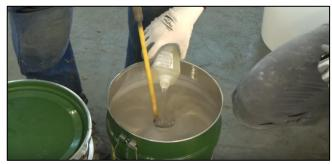
Figure 15. Mixing silicone & hardener component
