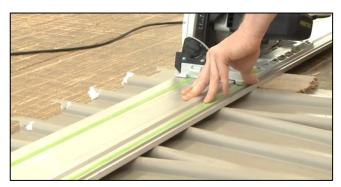
Figure 21. Cutting silicone
