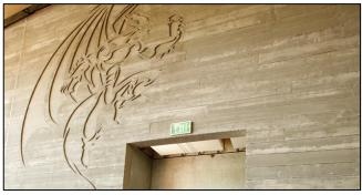
Figure 6. Negative patterns on concrete surfaces
