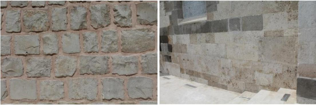
**Figure 3.** *Facade cleaning carried out on the mosque's east facade and north courtyard facade rough masonry stones*
