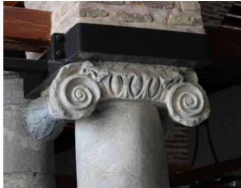
**Figure 8.** *Column headers after repair*
