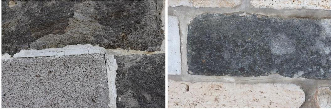
**Figure 13.** *Crack formation in joints due to thermal expansion*
