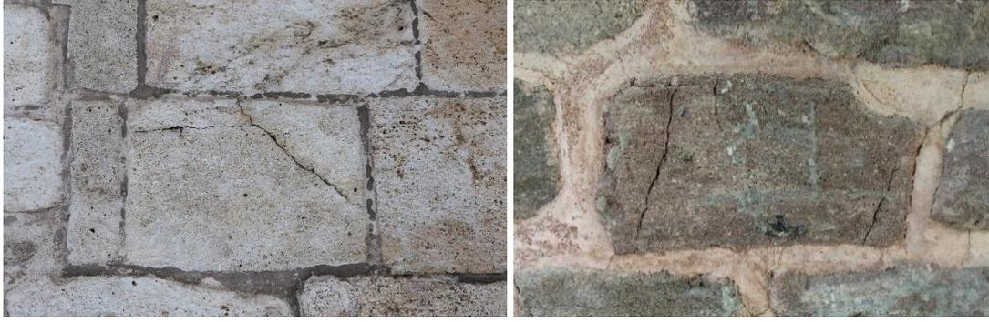
**Figure 12.** *Crack - fracture formations on the stone surface*
