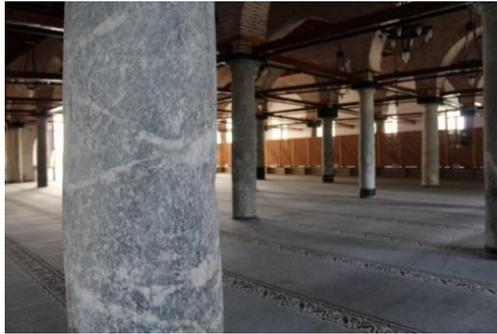
**Figure 7.** *Surface cleaned marble columns*
