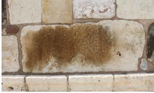
**Figure 15.** *Abrasion on stone surface due to chemical effects*
