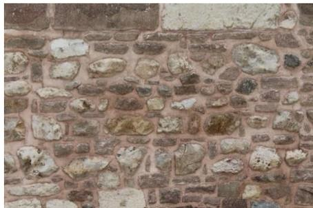
**Figure 5.** *Grouting with hydraulic lime added horasan mortar*
