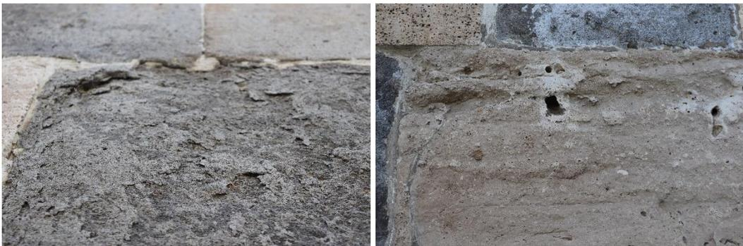
**Figure 17.** *Abrasion on stone surface*
