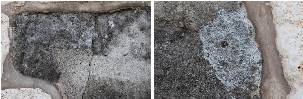
**Figure 14.** *Defects caused by air pollution and exhaust gases*
