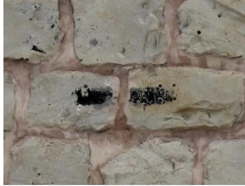
**Figure 18.** *Pollution caused by paint and similar marking tools*
