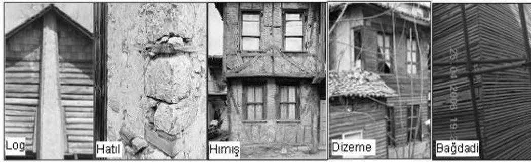
Figure 1. Types of wooden structures
