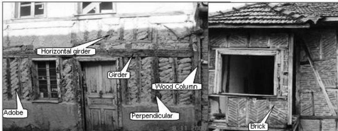
Figure 2. Details of a himiş structure
