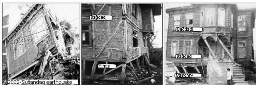
Figure 7. Earthquake damage at soft stories (Dogan 2007)
