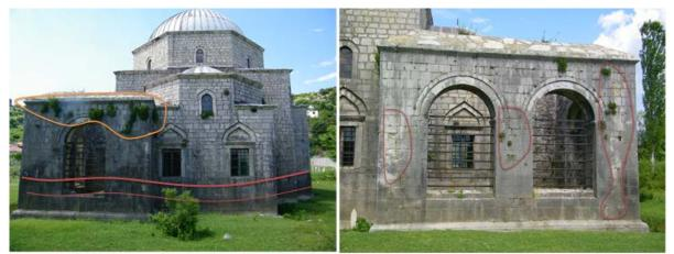
Figure 4. Traces of weathering factors influence and acceleration biological degradation in Lead Mosque
