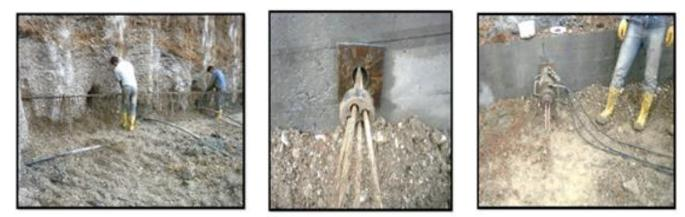
a) Phase3-Anchor and breast beam b) Phase3-Anchor Head c) Phase3-Prestressing Figure 10 Phase 3-Breast beam construction, placement of anchor heads, and prestressing at the site
