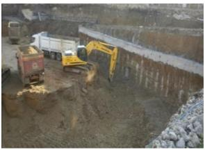
a) Phase 2-Plaxis 2D Model **b)** Phase2-Excavation up to the anchor level at the site **Figure 9**. Phase 2-Excavation up to anchor level and activation of bored piles
