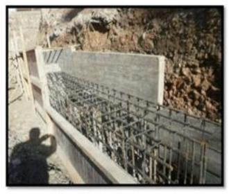
Figure 8. Phase1 Capping beam construction
