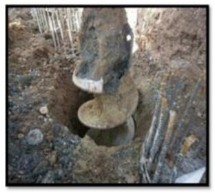
Figure 7. Phase 1 Bored pile construction
