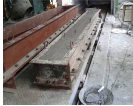
Figure 4: Casting of Beams
