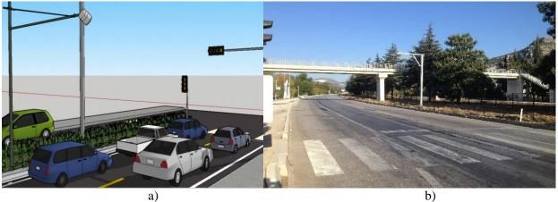
Fig.1. An example of a red light violation detection system (a) 3D design (b) real life application
