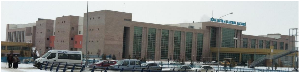
Figure 2. General view of the Erzurum Hospital
