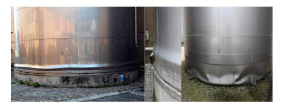
Figure 7. Elephant's foot buckling, Emilia earthquake, Italy, 20 and 29 May 2012 [13]
