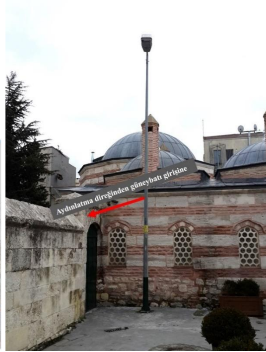
Fig. 8. Southwest corner of the courtyard.
