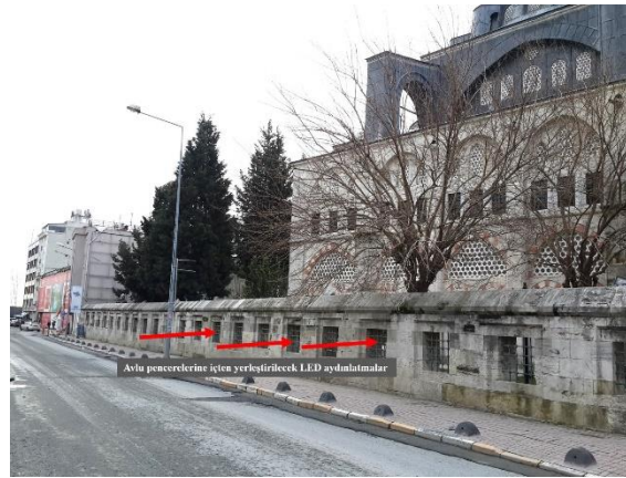
Fig. 9. Windows on the eastern wall of the courtyard.
