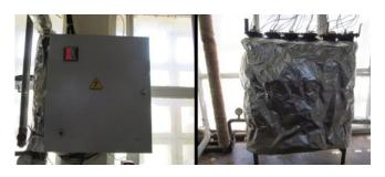
Figure 3. Electrical heater and its control panel.
