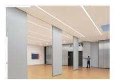
Figure 8. Sliding folding panel wall [7]
