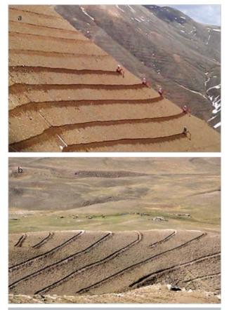
Figure 8. a, b. Contour terracing for erosion control (a) and improving soil moisture recharge and forage production (b) (GDCDE, 2015)
