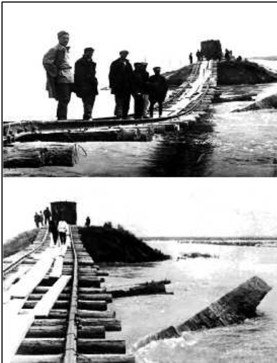
Figure.2 A part of the railroad damaged as a result of flood waters in 1915 (Pashayev and Hasanov, 2010)
