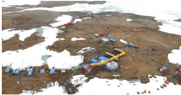
Figure 3. Syowa Station has 61 buildings and huts with two 300 kVA and a 200 kVA electric generators in 2013.
