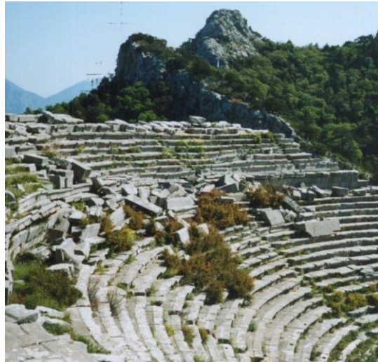
Figure 4. Traces of earthquake at Termessos (Güllük Dağı) theater.
