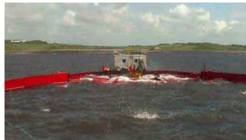
d. Wave Dragon system nearshore
