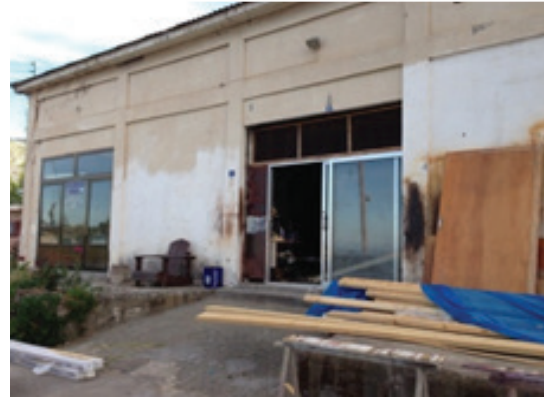
Figure 5. Ozanköy Olive oil mill, which currently works as carpenter (Eken and Varol, 2014)
