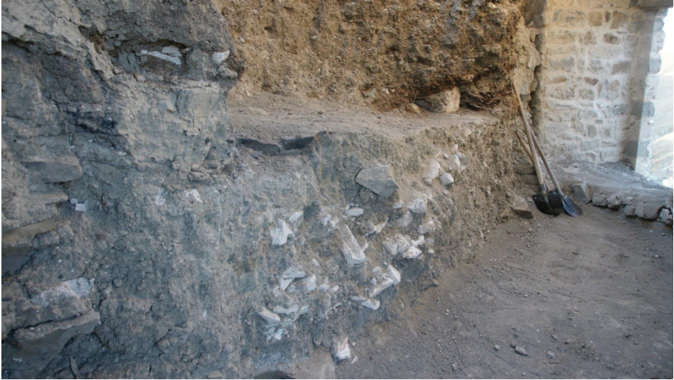
Fig. 3. Inside of the western tower (Excavation archive)
