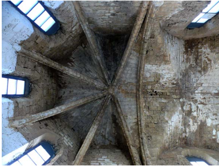
Fig. 4: Vaulting of apse of the Maronite Church of St. Anne, Famagusta. Photograph by Wilbert 'Skip' Norman
