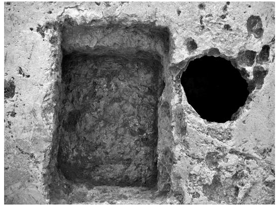
Fig. 18 Temple II, detail showing rock installations
