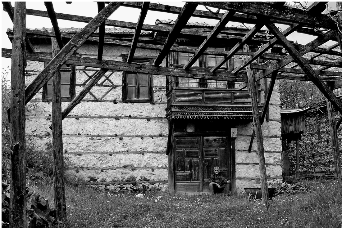
Fig. 6 The projections and characteristic masonry in the rural dwellings (Central district of Ürünlü).
