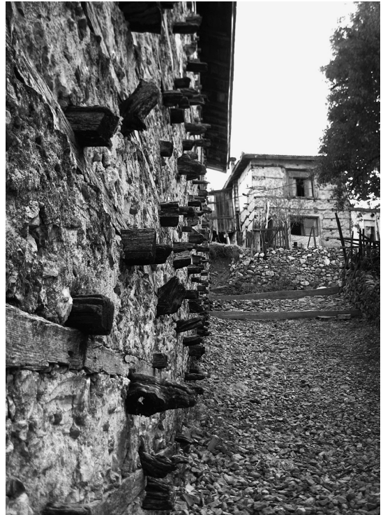
Fig. 4 The projecting tie beams ( peştivan ) constitute the characteristic spatiality of the traditional environment (Ürünlü).
