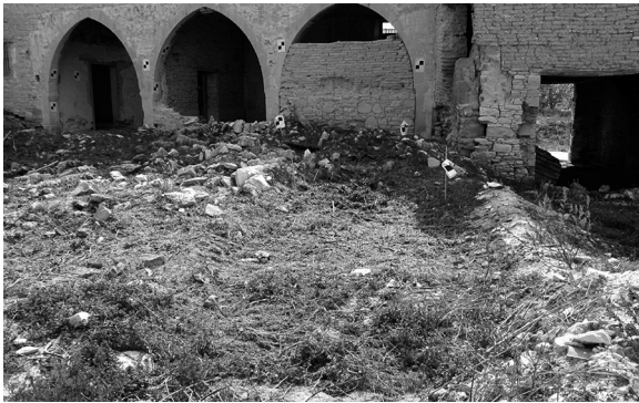
Fig. 14 Khan, destroyed Building B, view towards south onto north elevation of Building A; right: unassociated passageway, slight traces of walls of B under debris and vegetation
