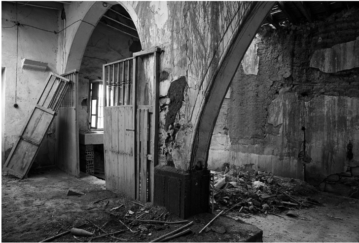
Fig. 12 Khan, Building G (coffee house), view from southern bay towards northern wall, souventza (cornice) on wall to left, middle pillar reinforced by concrete cover
