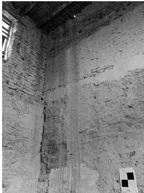
Fig. 13 Khan, Building A, view into south-west corner and of western wall of Room 3 shared with unassociated passageway
