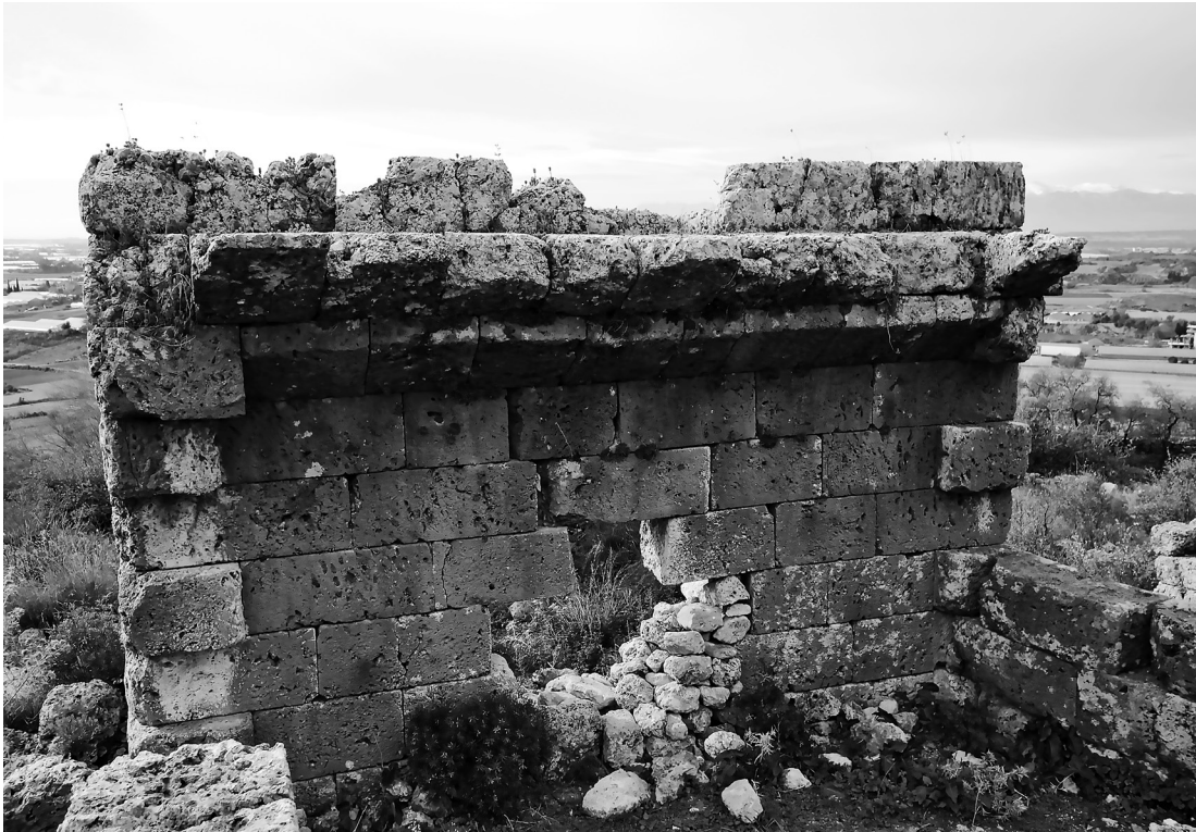
Fig. 14 Tower 1, epalxis on top of north wall
