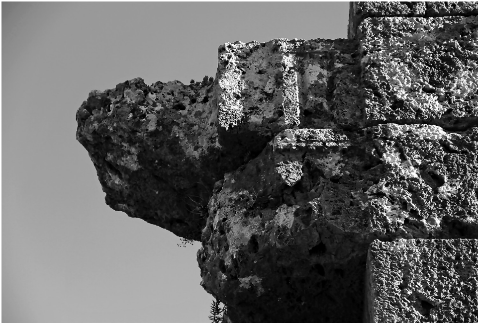
Fig. 10 Tower 1, Doric triglyph-metope fragment embedded in northwest corner
