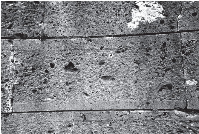
Fig. 2 Façade arrangement of isodomic wall of the complex's courtyard
