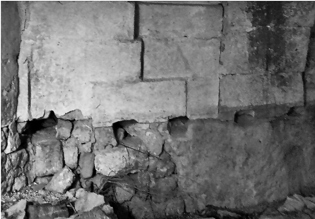
Fig. 8 Foundation type 1: Rock foundation
