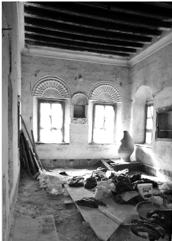
Fig. 24 Hezen of timber logs sitting on inner cornices
