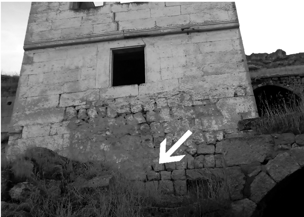
Fig. 12 Foundation type 4a: Deep-slope foundation
