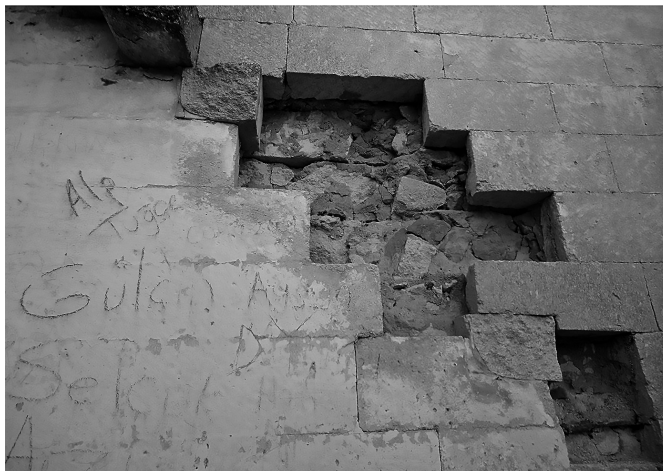
Fig. 17 Wall type 2: Thin, double- sided wall
