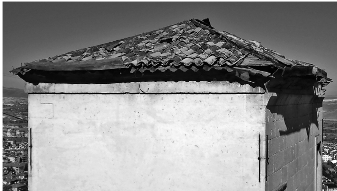
Fig. 16 Iron tie bars in first floor walls
