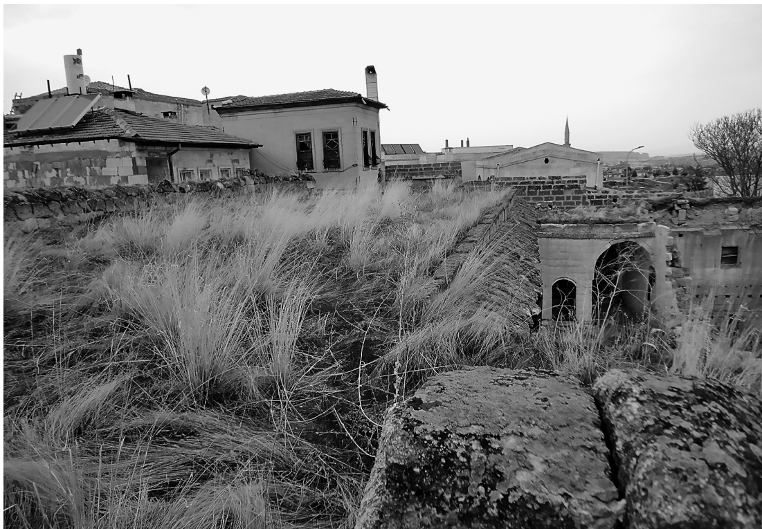
Fig. 26 Detail of earth roof
