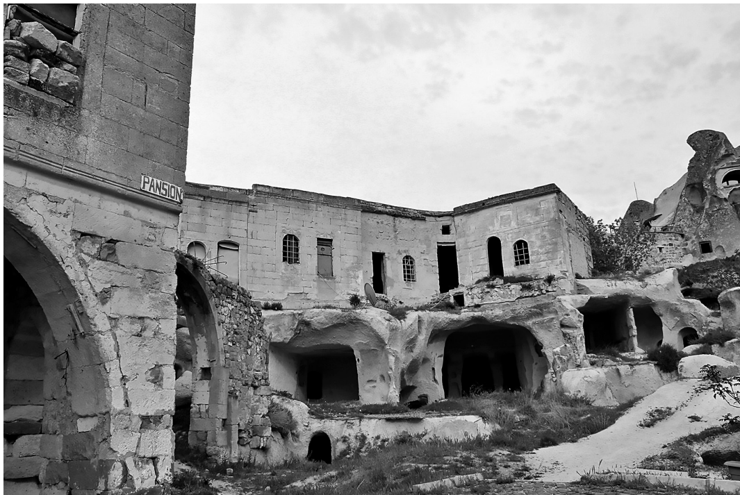
Fig. 4 Using rock-carved and masonry techniques together
