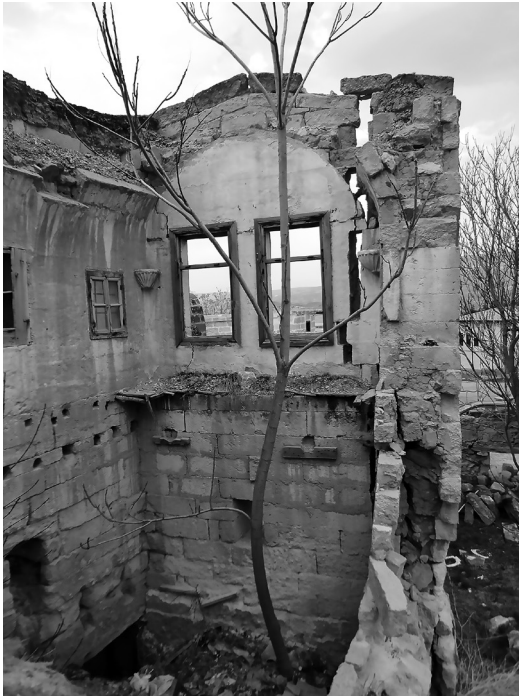
Fig. 18 Wall type 3: Thick, double-sided wall
