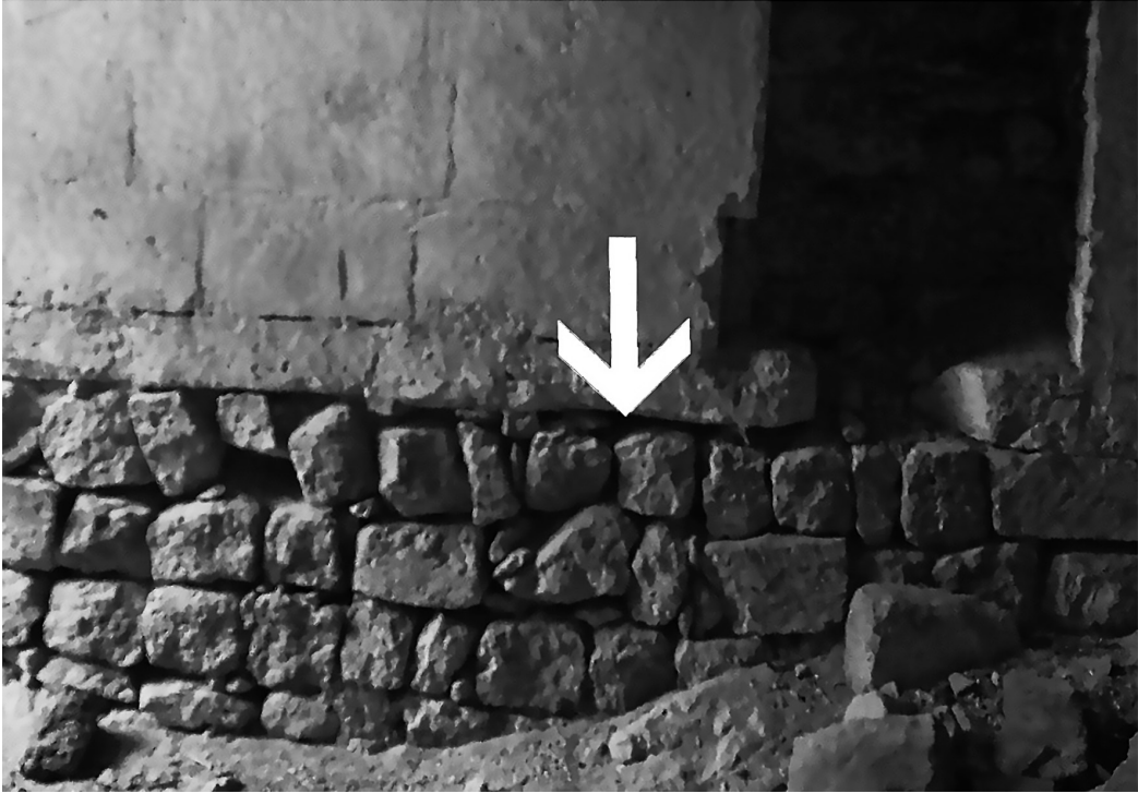
Fig. 13 Foundation type 4b: Deep-inner foundation
