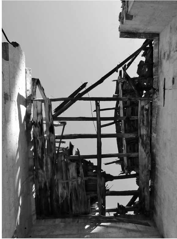
Fig. 23 Timber beams and ceiling coverings, bottom view
