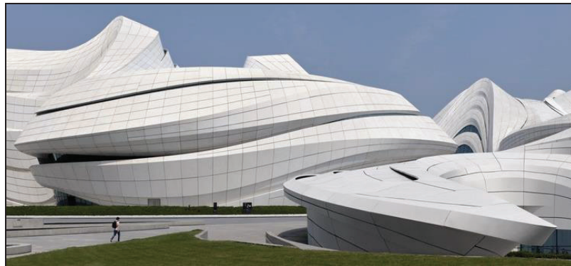
Figure 4. Cultural Center Changsha Shi, Zaha Hadid Architects, China Photo: Virgile Simon Bertrand
