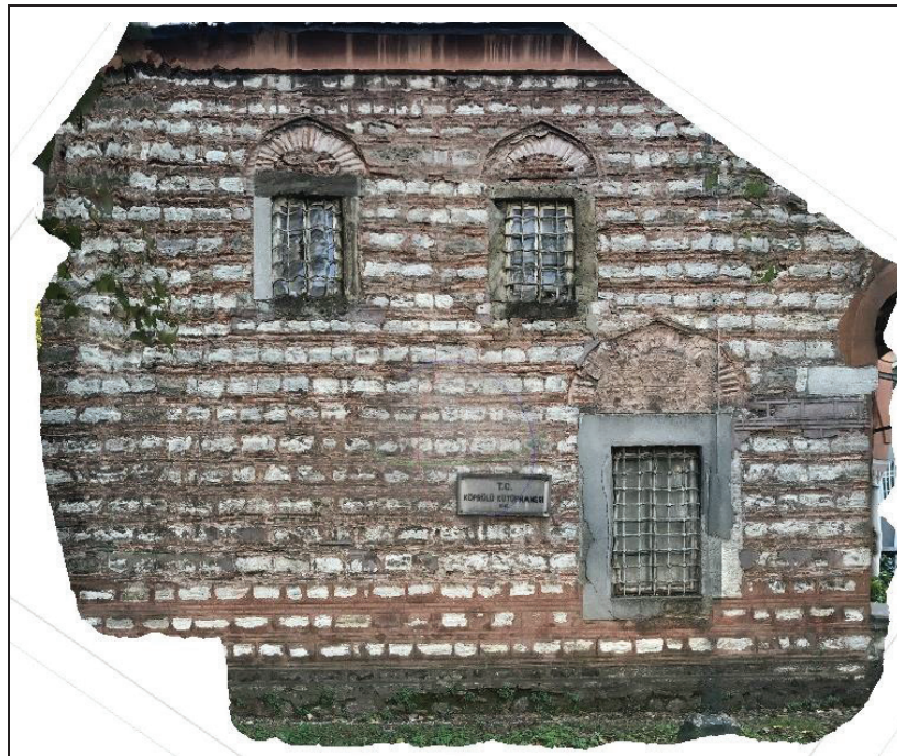
Figure 12. T.C Aydın University student study work The orthophotography photo of the Köprülü Library was formed by analyzing 394000 surfaces, 192000 intersections and pixels.
