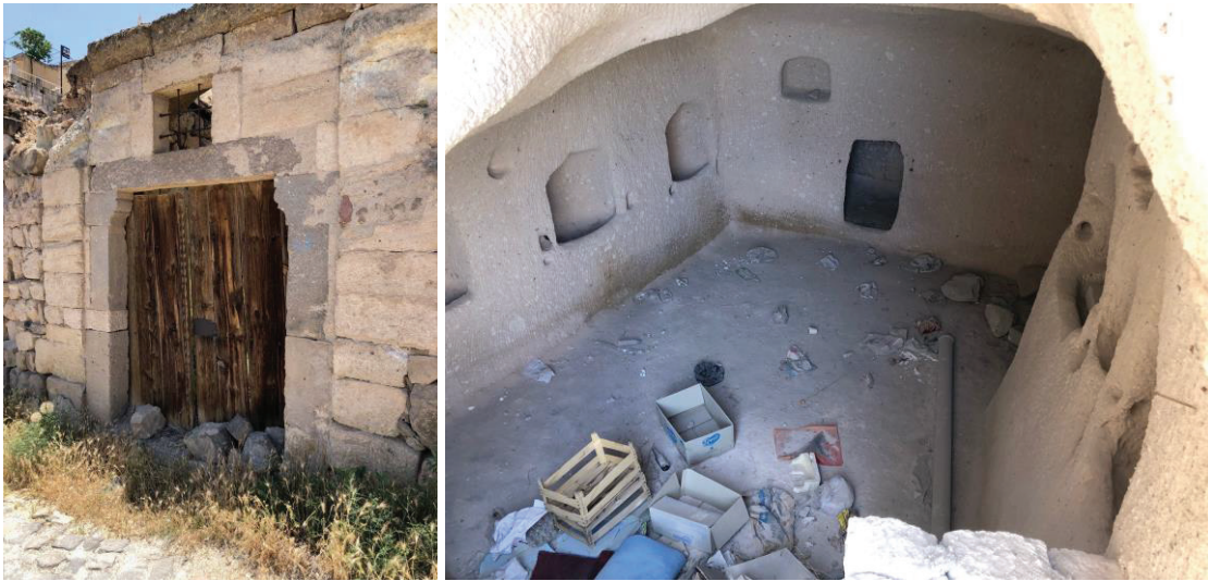
Figure 7. Two rooms and a small sofa on the upper floor or more rooms (Author photo archive 2019/2020)
