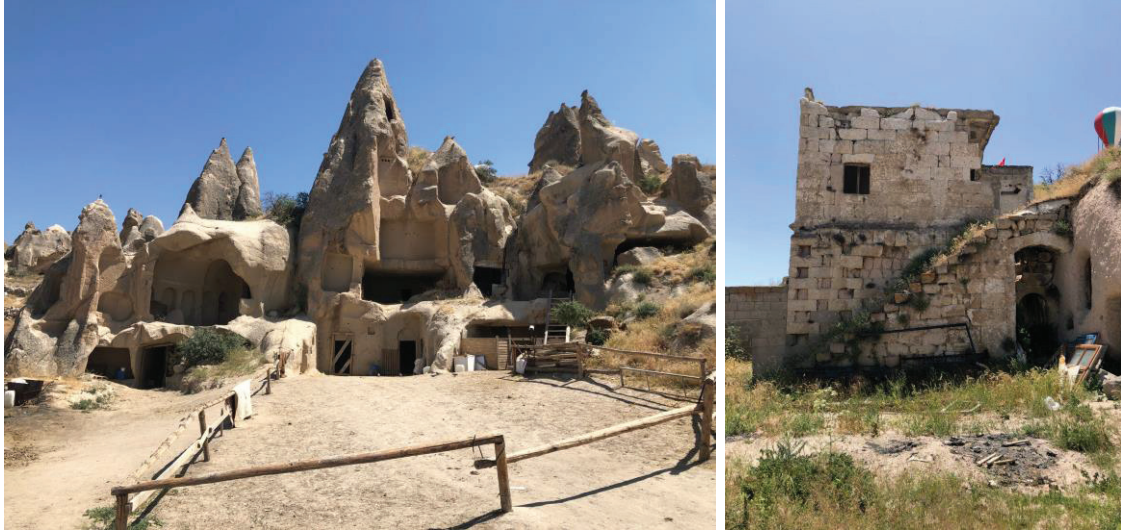
Figure 2. Rock carved housing example, Masonry housing example (Author photo archive 2019/2020)
