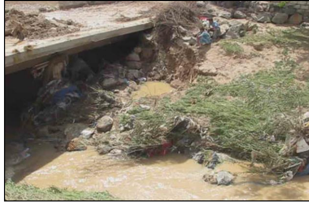
Resim 2. Rüşubat birikmesi yüzünden daralan kesit nedeniyle su köprü üzerinden akmış, taşkına sebep olmuştur. Şanlıurfa Boydere Köyü [5] (Photo 2. Because of narrowing cross-section with participation, the water had accrossed overcome of the bridge and had occured flood Şanlıurfa-Boydere Village [5])
