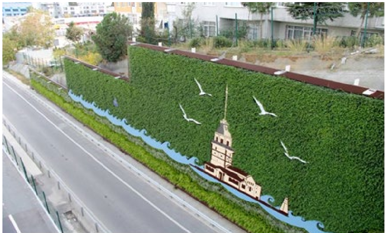
Fig. 4: Kadıköy, Eurasia Tunnel Exit Vertical Garden, Total Area: 610 m 2 [Url-6]
