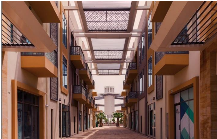
Figure 10. Shading elements and wind tower that made to prevent heating of the environment. (The Sustainable City, 2015)
