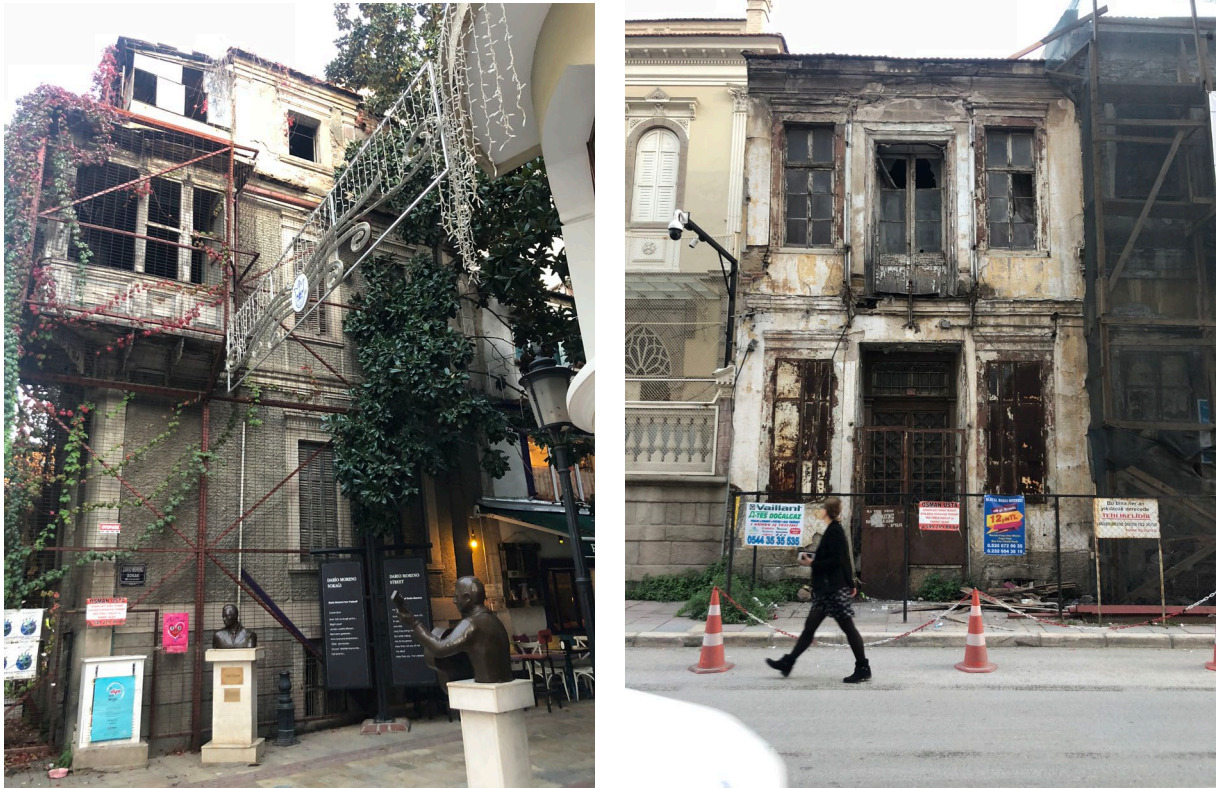
Figure 7. Historical abandoned houses
