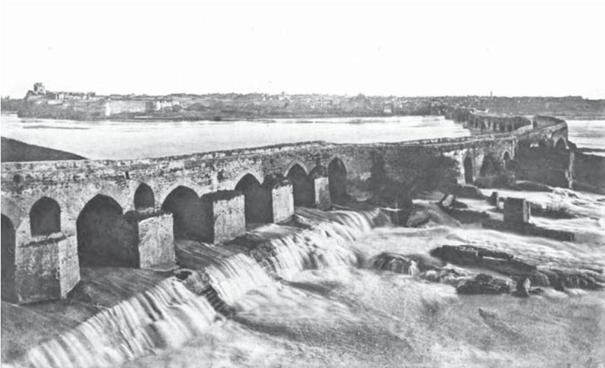
Fig.5. Photograph of Band-e Kaisar Bridge (pointed arches date to post antique restorations); M. Dieulafoy, 1884.
