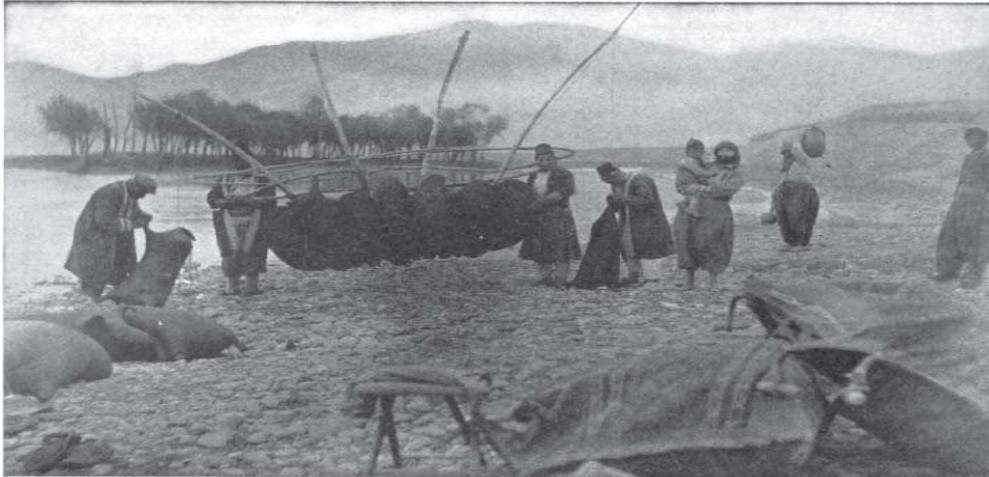
ARMENIANS CONSTRUCTING A RAFT OF INFLATED SHEEPSKINS ON THE BANKS OF THE EUPHRATES RIVER
