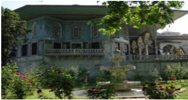
Figure 24. The Revan Mansion
