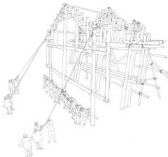
Figure 7. Erecting the structure, sketched by Ruchen Bian, Daili Village, 14/11/2016
