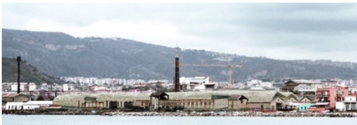
Figure 5. The new volumetric configuration in relation to the remains of pre-existing building
