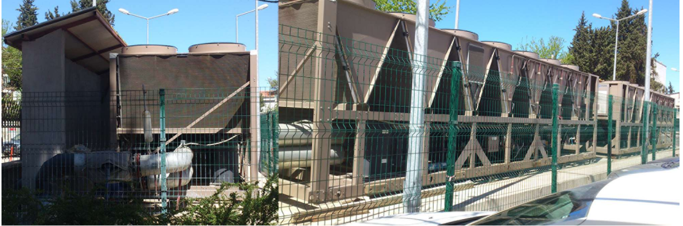
Figure 1. Air-cooled liquid chillers
