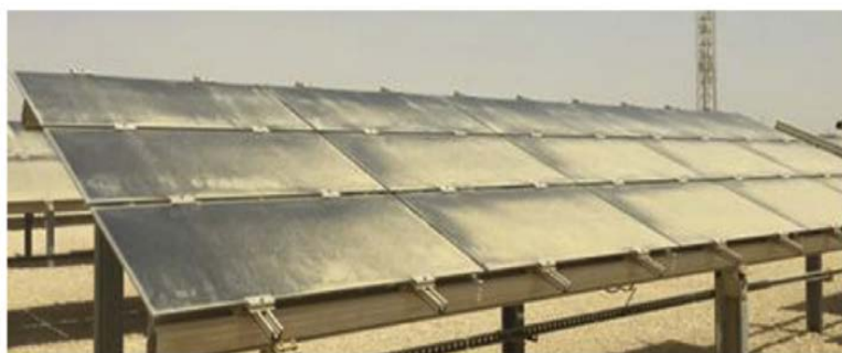
Figure 1 Soiled PV panels installed in Doha, Qatar [5]
