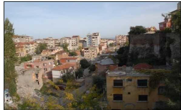
Figure 5. Buildings in Zagnos Valley before expropriation for urban regeneration
