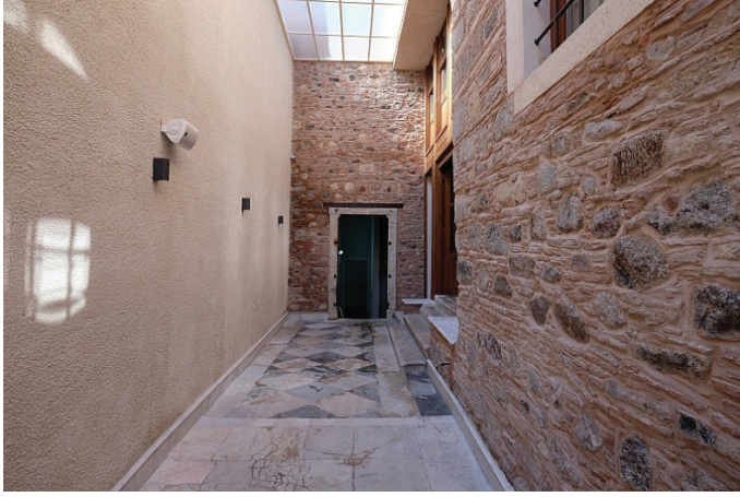
F. 19. Post-restoration, northern part of courtyard (Mehmet Yasa, 2018)
