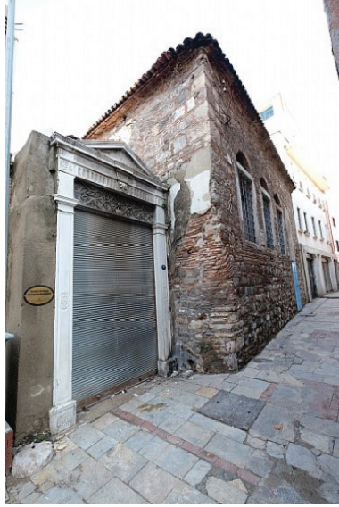
F. 2. Pre-restoration, southern façade and courtyard entrance (Mehmet Yasa, 2017)
